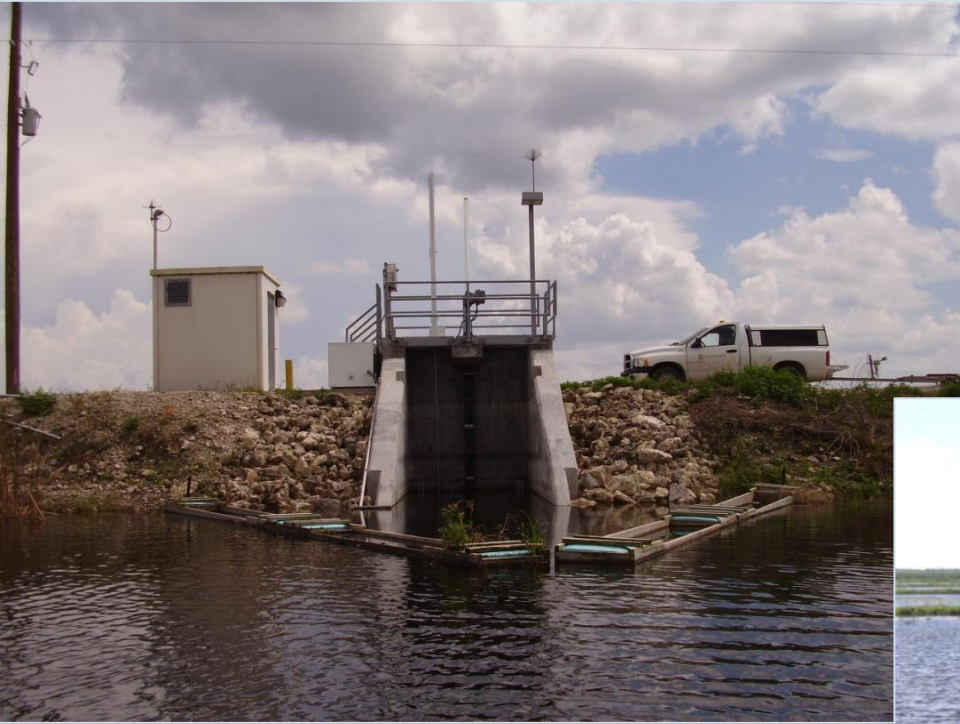
Upstream view of inflow structure
